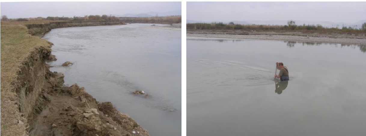
Figure 7.2: Osumi River and its eroding bank
